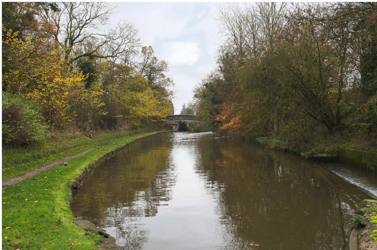
Figure 1: Shropshire Union Canal at Adderley
